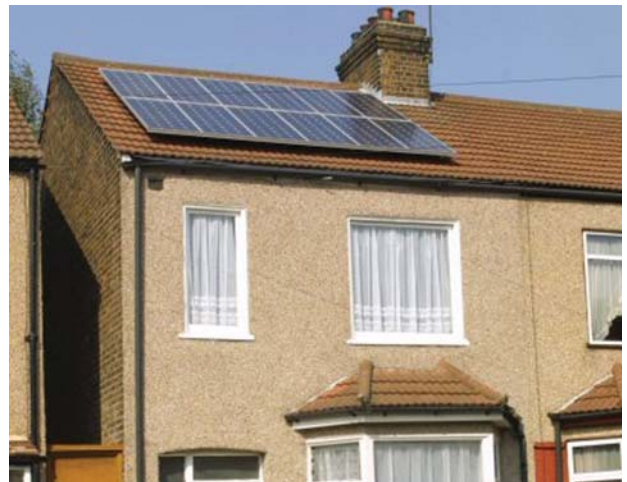
Photovoltaic installation (photo courtesy Energy Saving Trust)
