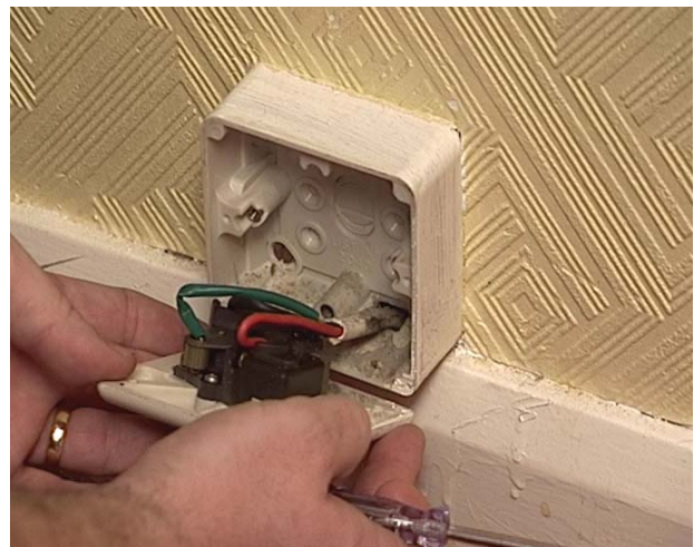
Inspecting a socket-outlet
