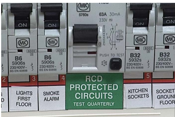
RCD in typical split load consumer unit
