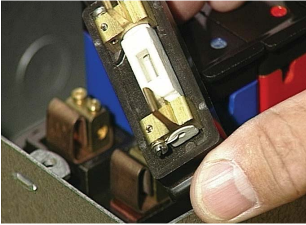
Checking a fuse carrier
